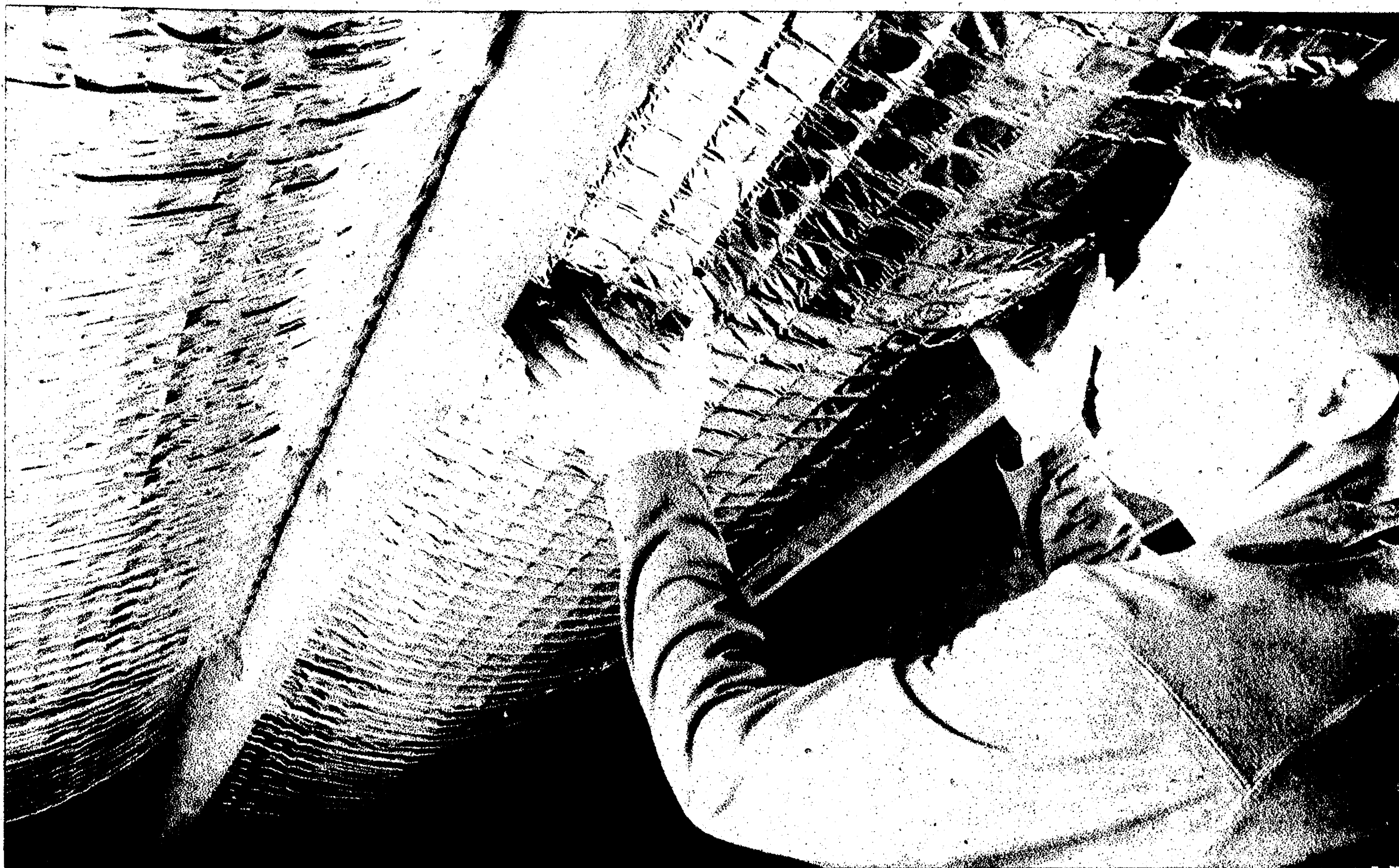
Energy Star-approved Enerflex Radiant Barrier, which reflects up to 96 percent of the sun's radiant energy and helps cool attic space up to 30 degrees, is easy to install and qualifies for a tax credit for savings up to $1,500.
