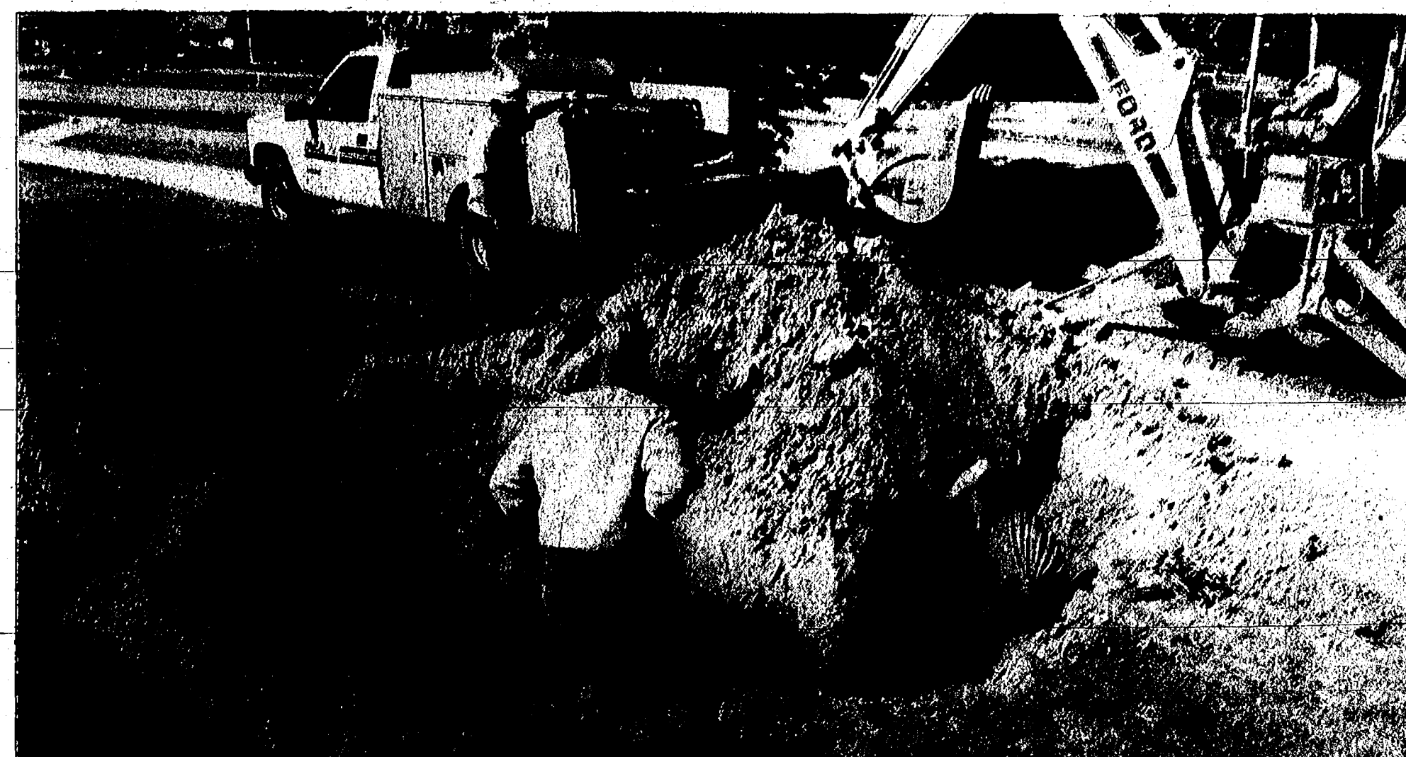
MichCon workmen finish pinching off a ruptured gas main at M-52 on Sept. 8, and begin to rebury it. The ruptured main led police and the Fire Department to evacuate the area and divert traffic for two hours.
