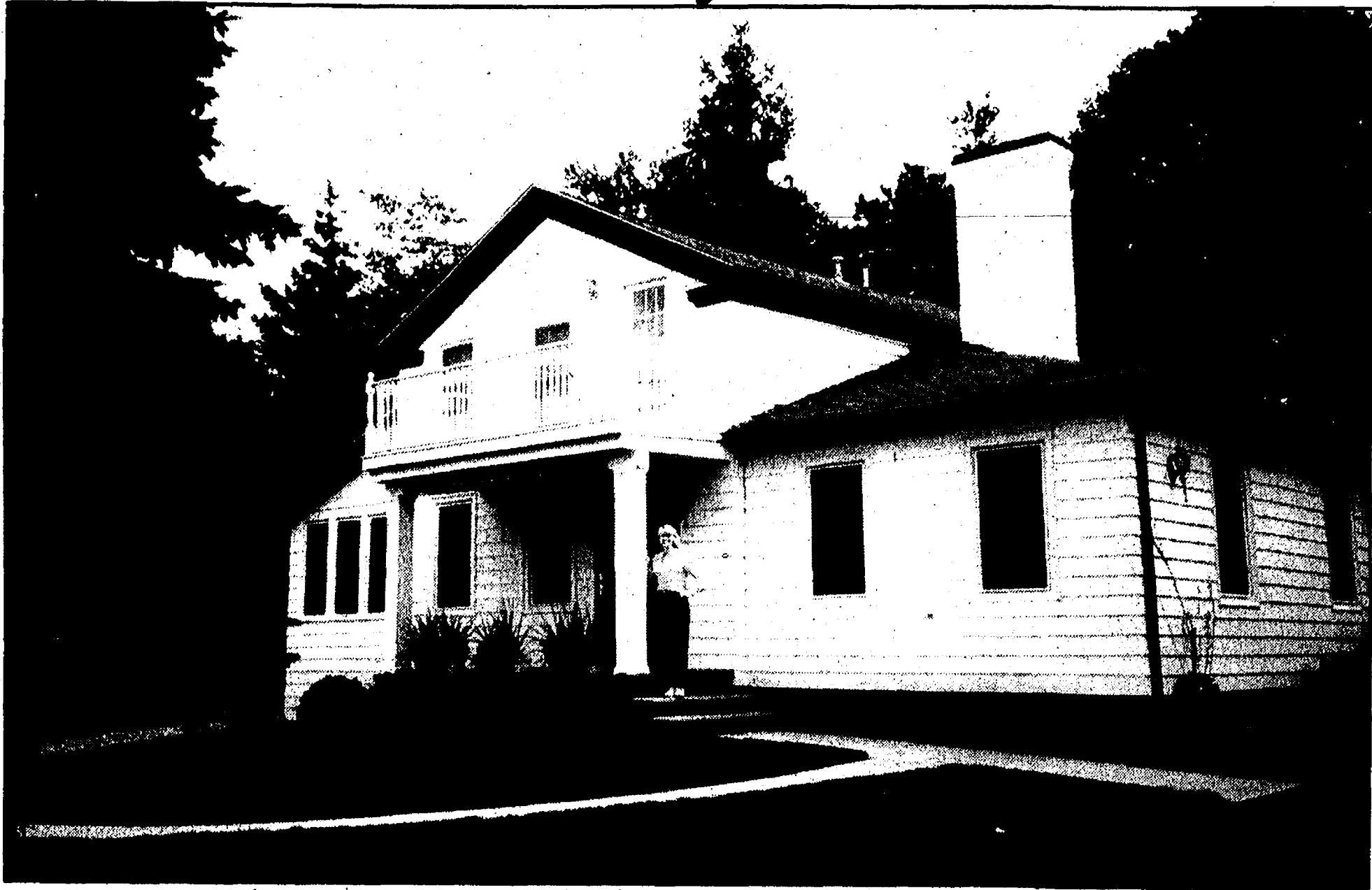
Remodeled for Glenda Warner's law office, the back of the house, known as the Mial Boyd house, is now the front with a new porch and balcony facing north toward the train depot.
