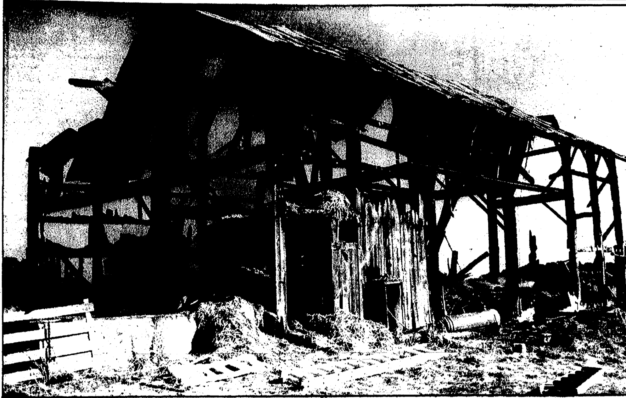
An accidental fire destroyed this 100-year-old barn at 12165 Trinkle Road Friday night for an estimated $50,000 damage. The homeowner's son and two of his friends were smoking in the barn
