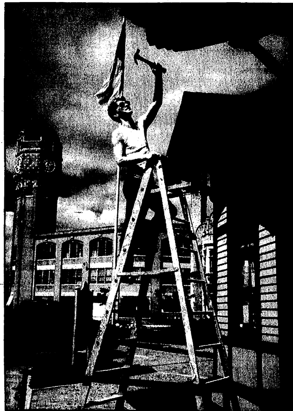
Dave Lukasiac, a board member of the Chelsea Depot Association, is pictured repairing the damaged overhang.
