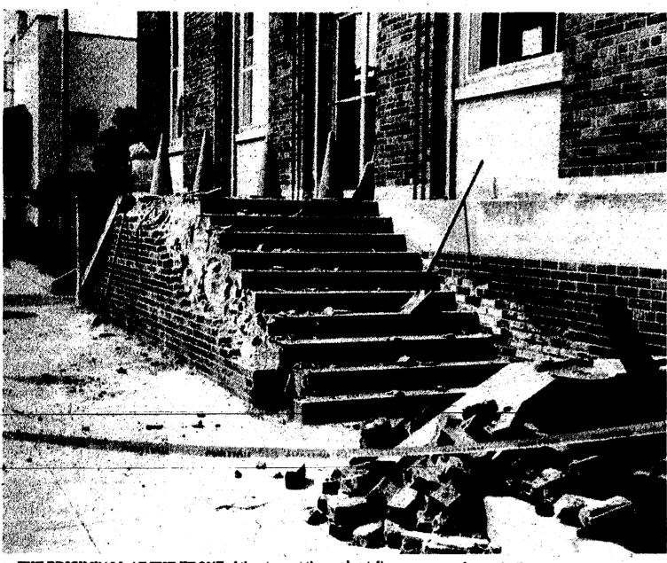
Chelsea Post Office is being replaced. Water seeped Larry Williams hopes the problem will be solved perbehind the wall, causing it to crack. The wall was replaced manently this time.
