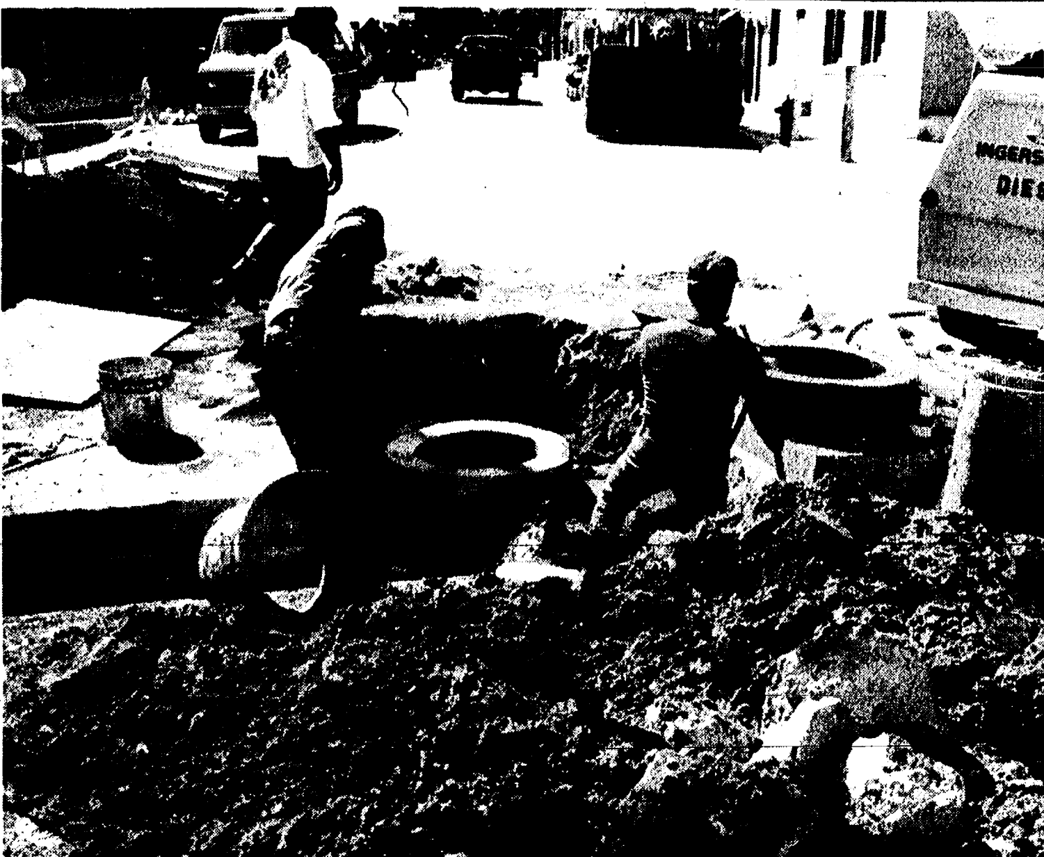
A MANHOLE has been installed where soil washed away under M-52 due to a crack in the storm sewer line. The manhole will allow easier access to the line. Crews discovered the void under the road as they were cutting
