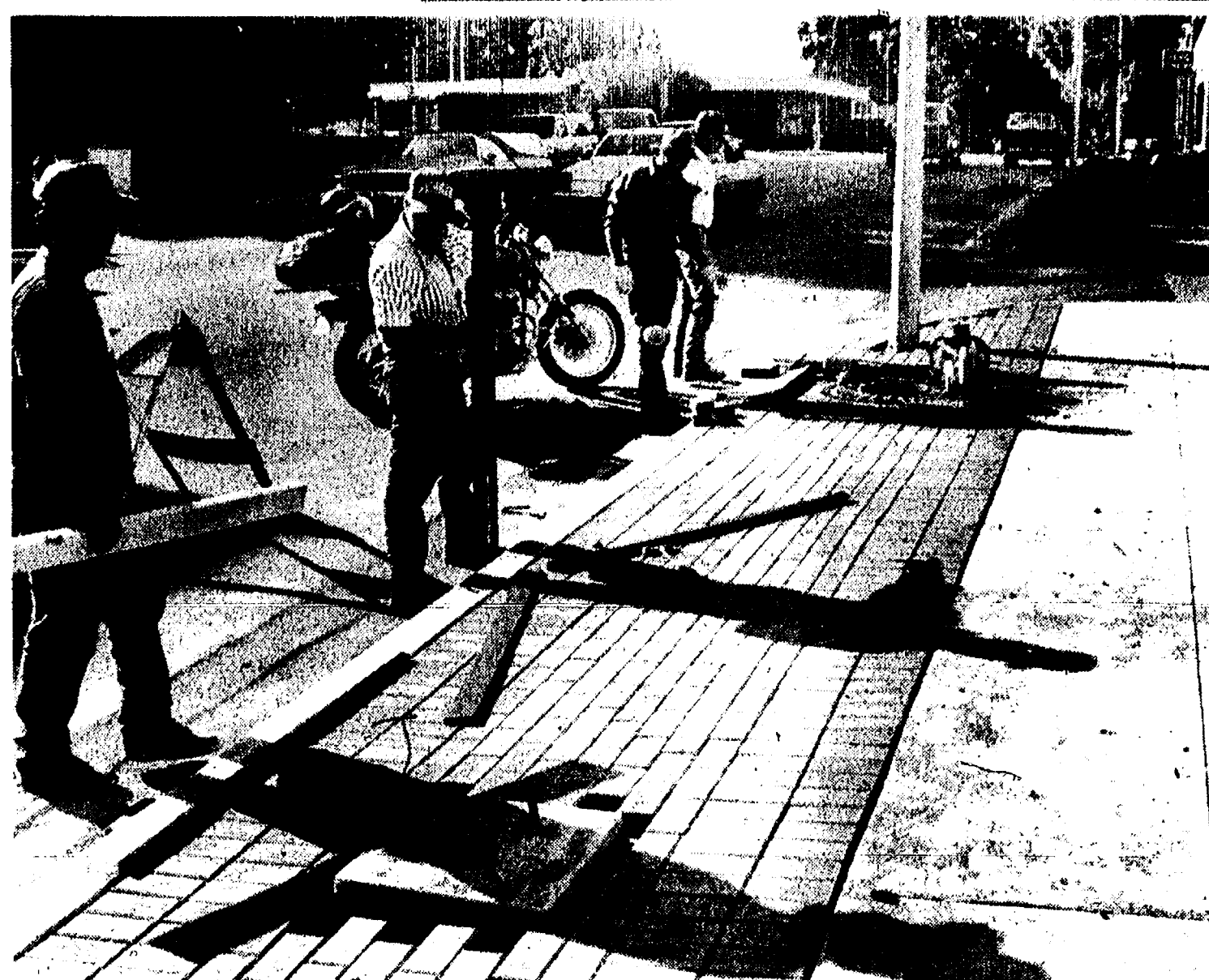
BRICK PAVERS are being installed along Main St. as streetscape project. The pavers resemble antique brick part of the Downtown Development Authority's but are actually colored concrete blocks.
