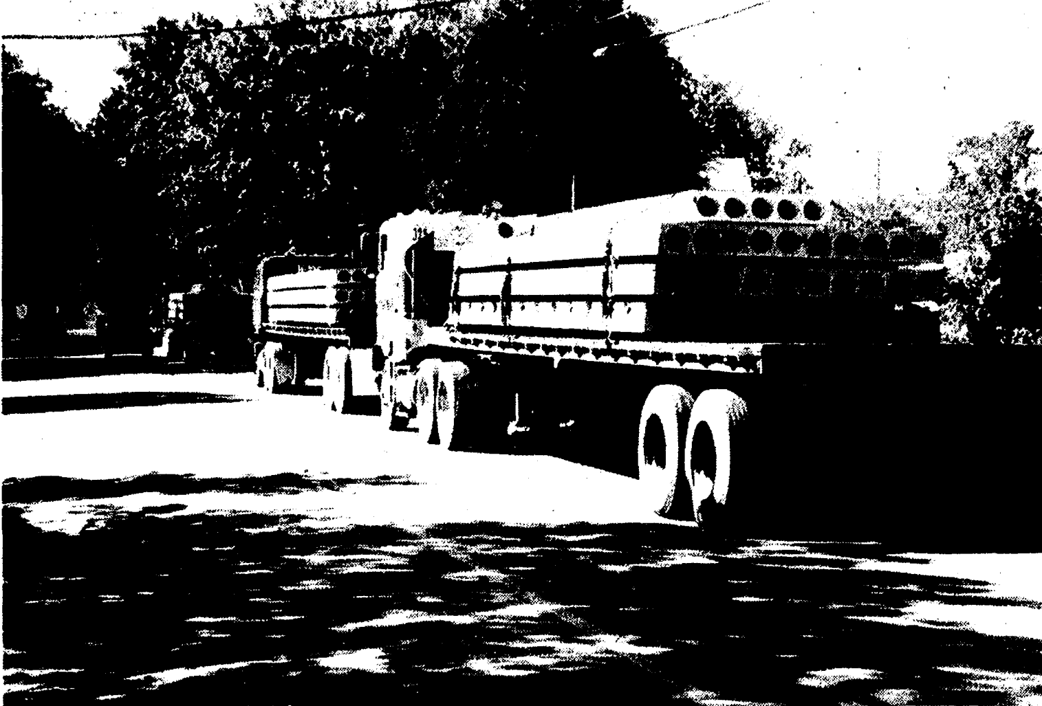
CONCRETE CASTINGS ON TRUCKS lined up on W. Middle St. on Monday are being used to construct the floors at the new Chelsea United Methodist Retirement Home facility. The holes in the castings are made to keep the weight down. The contractor said the panels, due to their method of construction, have been shown to be stronger than solid concrete. The panels are lifted into place by crane.
