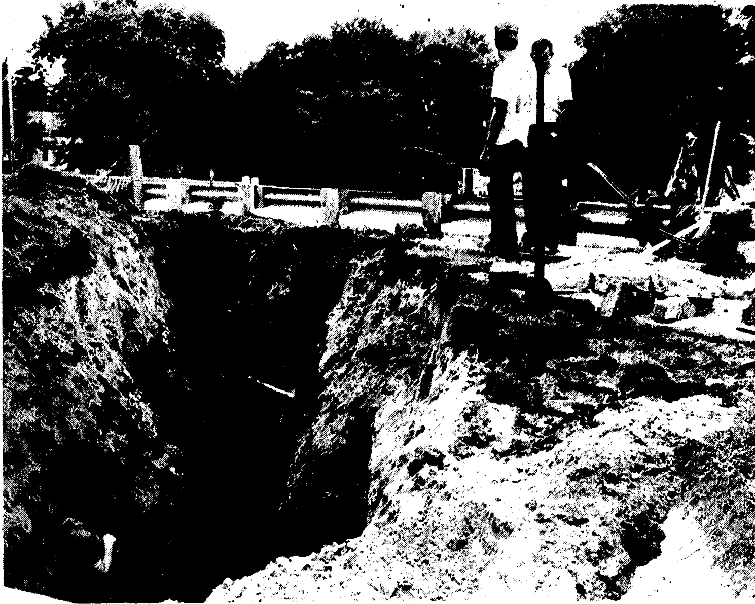
A NEW SEWER LINE has been tunneled under N. Main St. from Veteran's Park onto property owned by Art and Ruth Dils on N. Main St. The new line will also eventually require that Letts Creek be dammed up temporarily so that sewer line can be placed underneath.
