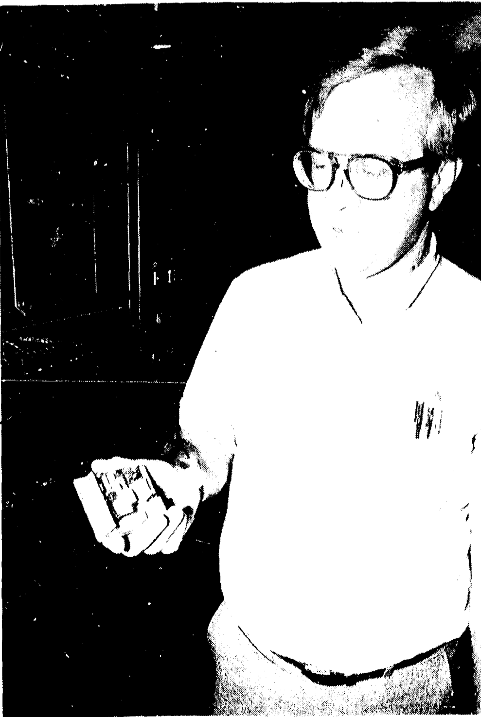
MICHIGAN BELL recently finished installing $1.5 million in new digital equipment at its W. Middle St. building. Above, chief switchman Leonard Cieciek holds the circuitry necessary to handle one telephone number in the 475 exchange.
