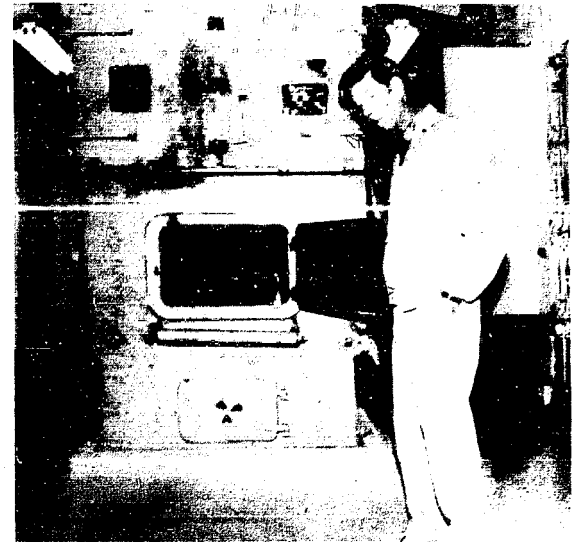
WOOD ENERGY will be used to heat the building and provide hot water for the 80 inmates in the new facility, explained CLTS staff member Bill Frame. Approximately 1,000 pounds of wood a day will be used during the winter, Frame said.
