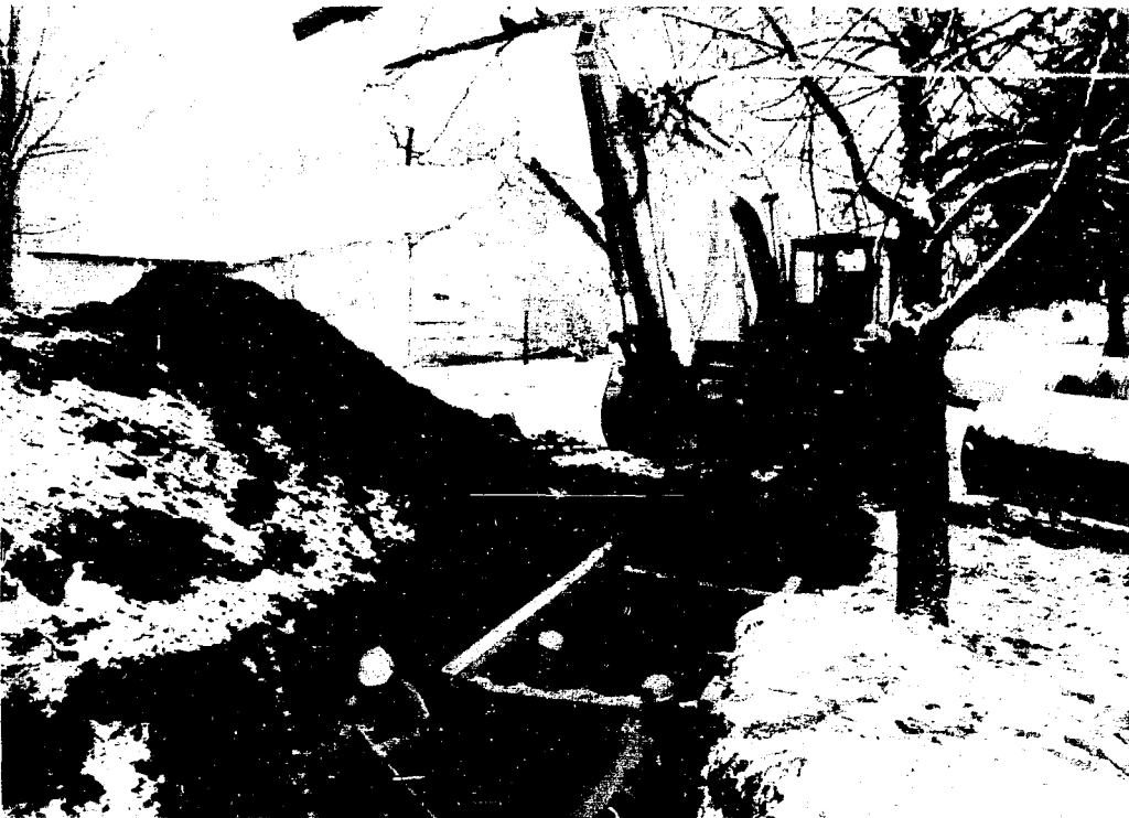
A SECTION OF STORM SEWER near Grant and W. Middle St. is being replaced by village crews this week to alleviate some of the problems caused by heavy rains. Above, village workers, guided by
