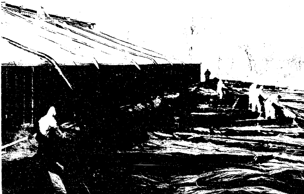
PREPARING THE TARP to go over the corn storage bin at Honeggers on Dexter-Chelsea Rd. are company workers. The one-piece tarp, designed specifically for the 175' by 70' bin, was hauled over the bin against the wind by heavy ropes. It will protect the corn
