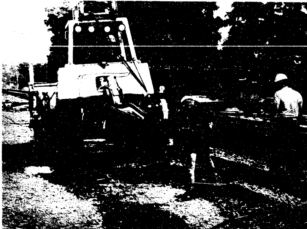
UNDERGROUND COMMUNICATIONS cable was installed by Conrail workers last week as scheduled maintenance on the tracks continued. The hole was dug and cable laid simultaneously.
