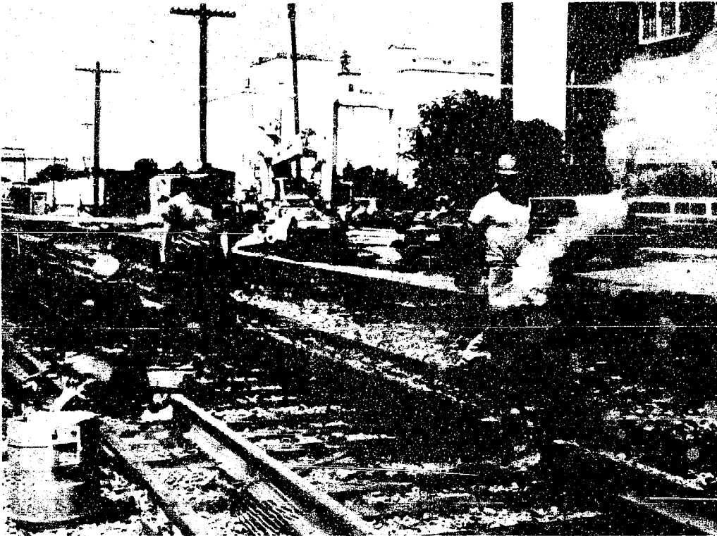
CONRAIL "WELDING CREW 311" placed the crucible atop a new section of rail (shown at the left in the photo) installed near The Chelsea Standard offices late last week and stoked a fire to weld the section in place. Intense heat and brilliance from the special welding process developed in the early 1950's by rail crews in France was
