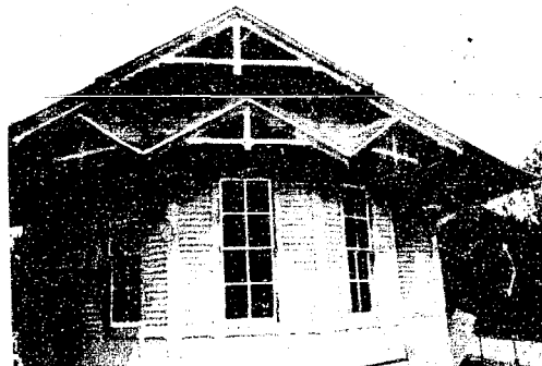
WEST END OF DEPOT with newly installed windows also contains newly crafted reproductions of ornamental woodwork. Other replicas of deteriorated or damaged ornaments are yet to be installed.
