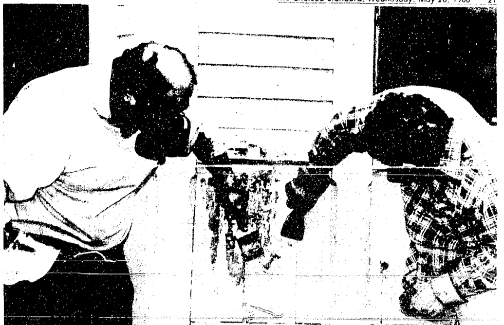
CHARLES SHIVER, left, joins with Denny Howard, in scraping layers of liquified paint from the wood surface of the Chelsea depot. The paint has been made to rise from the surface of the wood with a propane gas torch at a temperature somewhat above 600 degrees
