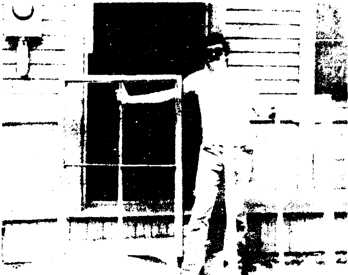
ORIGINAL 1880 WINDOW FRAMES from the Chelsea depot are displayed by Bob Colling of Shiver Restoration. Each frame has been stripped down to the bare wood and gouged to accommodate modern double pane insulating glass. The
