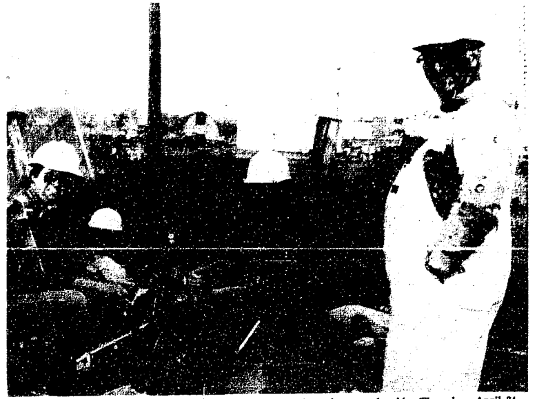
MICHIGAN BELL SPLICING TECHNICIANS Fred Lindsay, Dan Garrett, and Len Minnebo work as a team to match tiny pairs of lines and correct the chaos left after a Conrail construction crew doing work on a signal accidentally severed a
