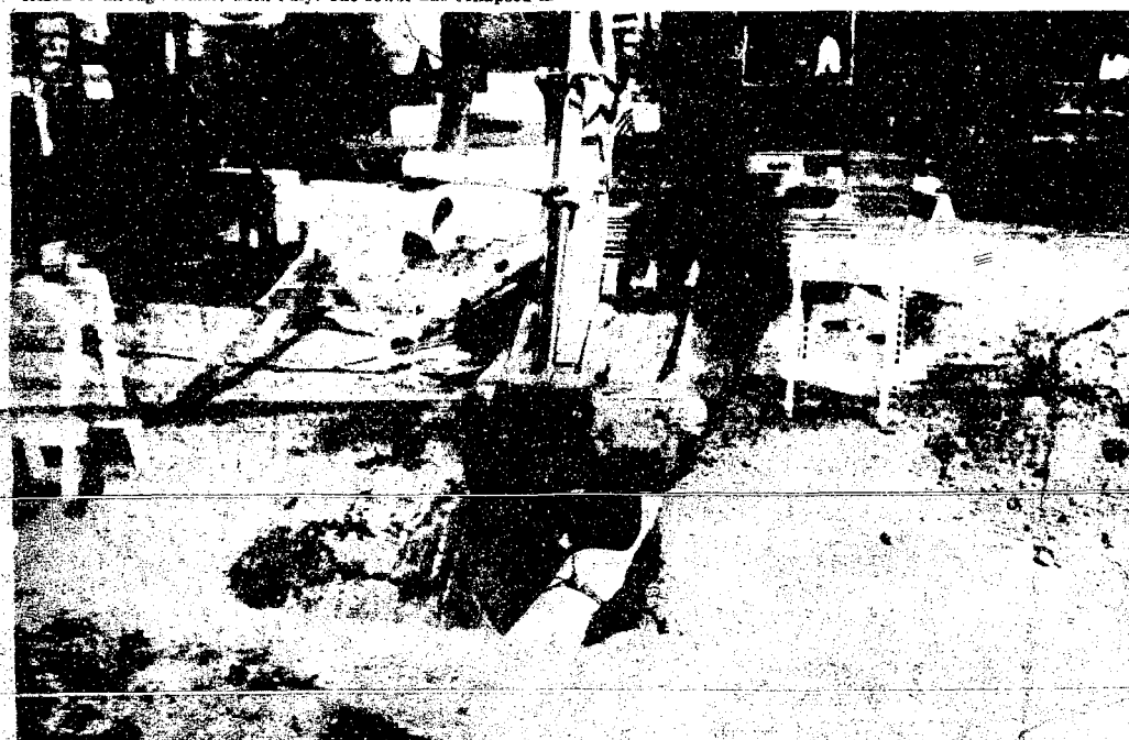
DROPPING IN THE PIPE for the new storm sewer on W. Middle St. is heavy work and takes careful positioning. Village workers began construction last Friday of 200 feet of storm sewer, a job that is expected to take more than two months and more than 800 manhours of village labor.
