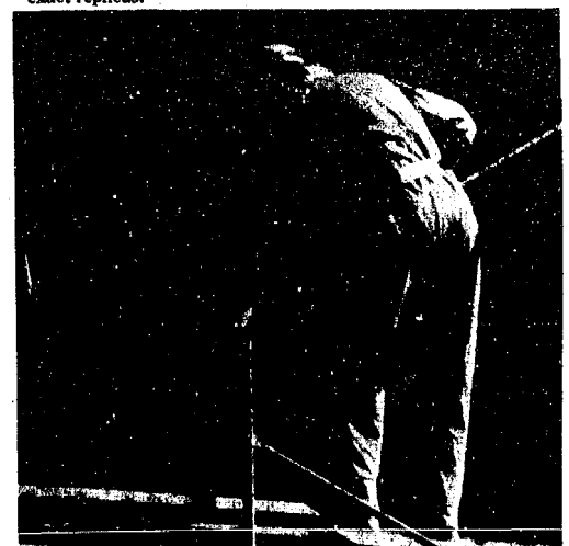
ROD SWEENEY, on scaffold, removed metal piping that was used as a conduit for electrical wires from underside of the roof. The pipe could not have been part of the 1880 building since Thomas Edison had invented the incandescent electric lamp just the year before.
