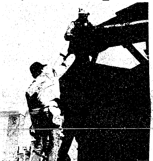
TIMBERS DAMAGED at the southwest corner of the depot roof are being removed by Jim Bauer (top) and Jerry Barth. Damage was believed done by a truck with an extra high trailer.
