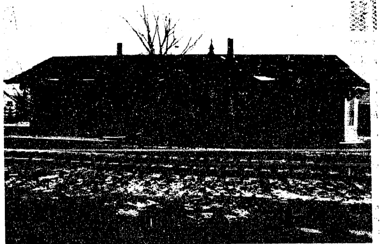
PROFESSIONAL REPAINTING OF THE DEPOT is expected to start in April, beginning with a thorough removal of paint layers applied from 1880 to 1984. Researchers believe that the original colors for all Michigan Central stations was gray with a forest green trim. The expert paint removal process will tell.
