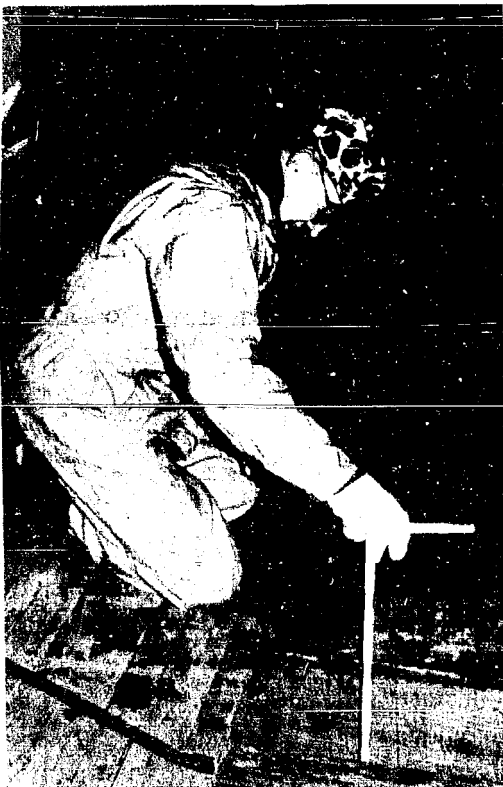
WITH A FOLDING RULE, Architect Lindauer measured the depth of the crawl space beneath the old rail station. He determined that there is ample room for the installation of heating and air conditioning ducts.
