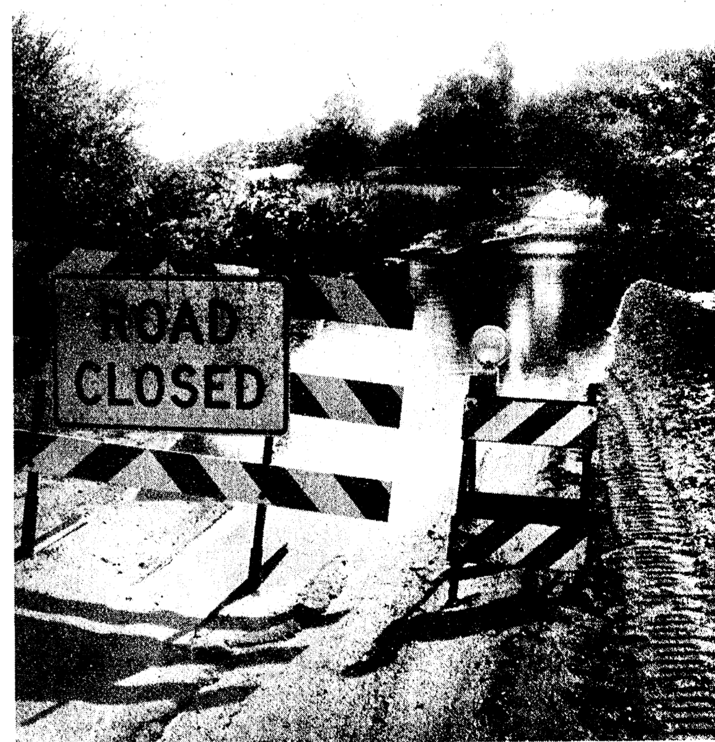
TRINKLE RD. between Freer and Fletcher Rds. is closed to through traffic because of flooding. County road engineers say the problem is caused by deep muck soil where Trinkle Rd.
