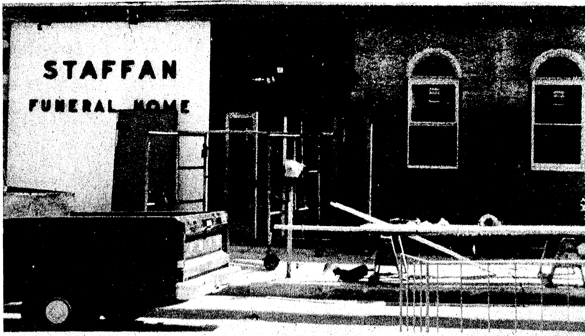
A FACELIFT is being given to the Staffan-Mitchell Funeral Home on Park St. The entire front of the building is being changed, including the foyer. New windows and a new front door have been in-
