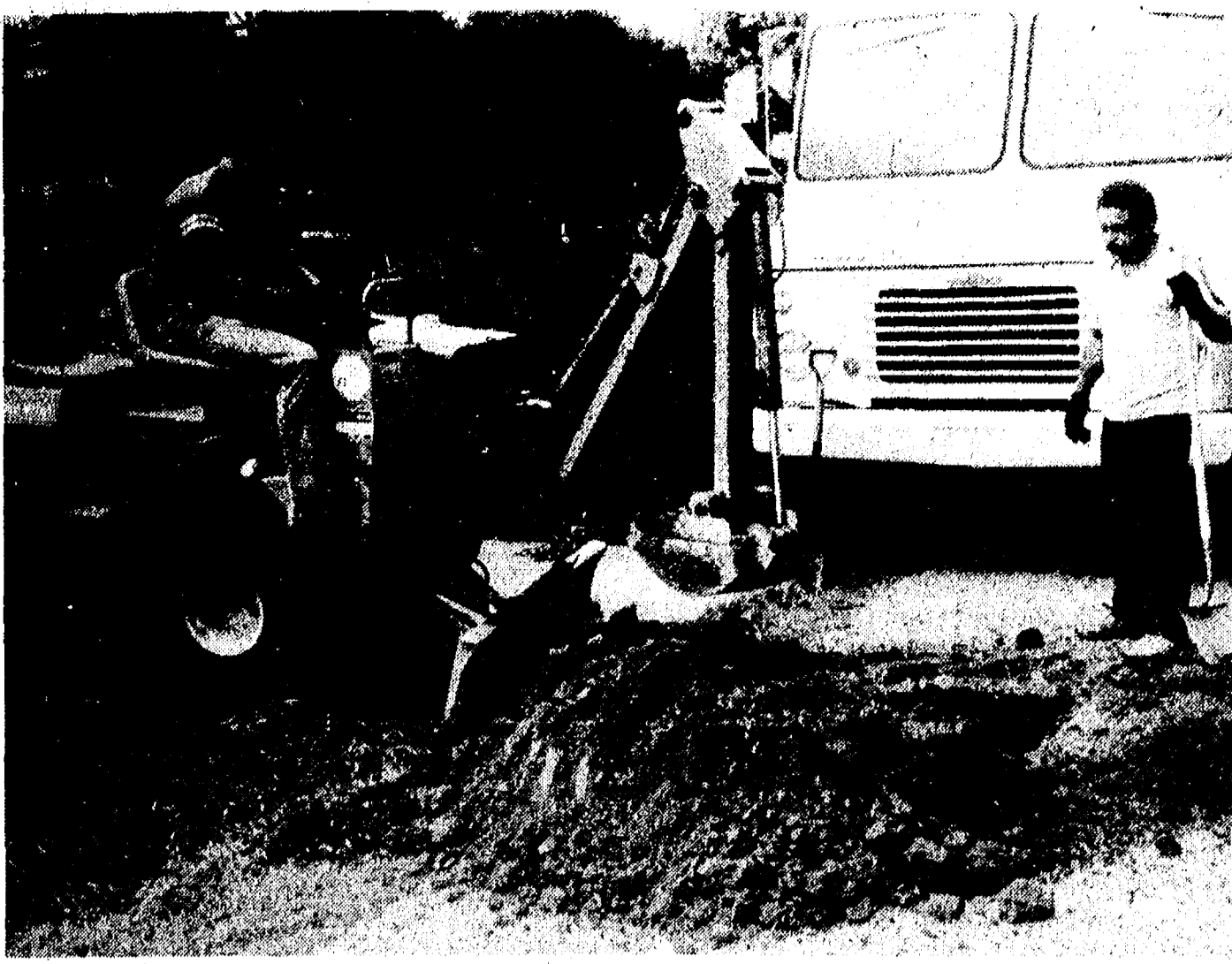
GAS SERVICE LINES REPAIRED: A Michigan Consolidated Gas Co. crew has been repairing service lines in the village during the past week. The work involved fixing small underground leaks. Shown excavating a hole on Railroad St. are Bob Murphy (left) and Mike Otto.
