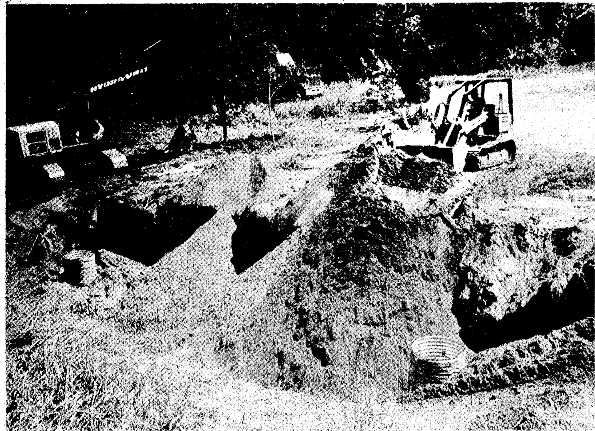
CONTAMINATED SOIL REMOVED: About 1,000 cubic yards of gasoline-soaked soil has been removed from in and around a drainage ditch south of the Mobil station on S. Main St. Some 4,000 gallons of gas were spilled during a hostage-taking incident on Aug. 5.
