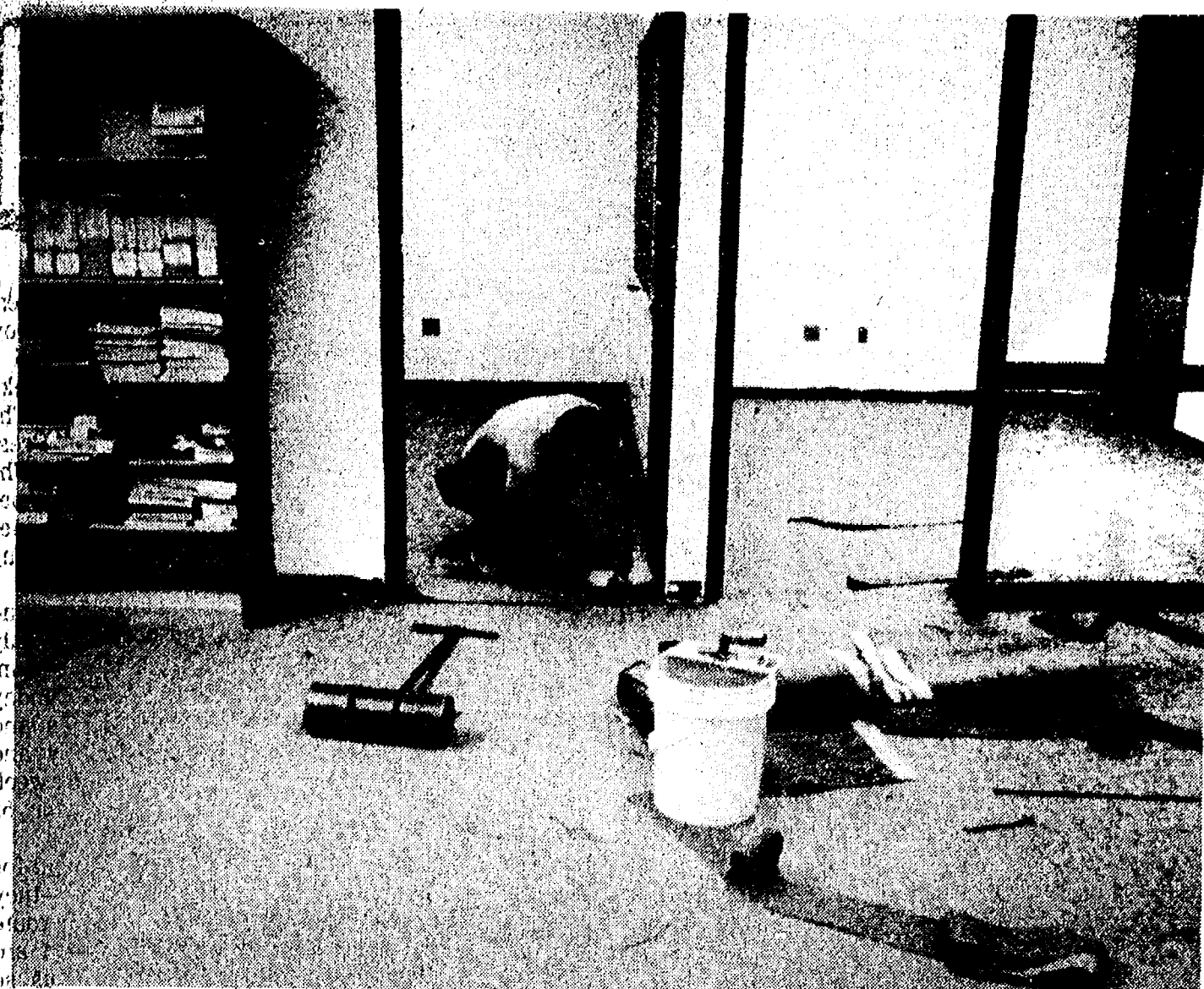
THE MIDDLE SCHOOL LIBRARY will have a little different look this fall as workers recently finished installing brown carpet over the existing tile in the main library, the adjoining conference rooms, and the librarian's office. Earlier this summer the walls were painted a slightly lighter color.
