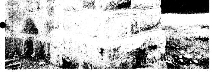
CONCRETE CAP IN PLACE: This is one of the néw concrete pillar caps formed from a handshaped plywood mold. Its curves, grooves and lines are perfect. The stonework at the bottom of
