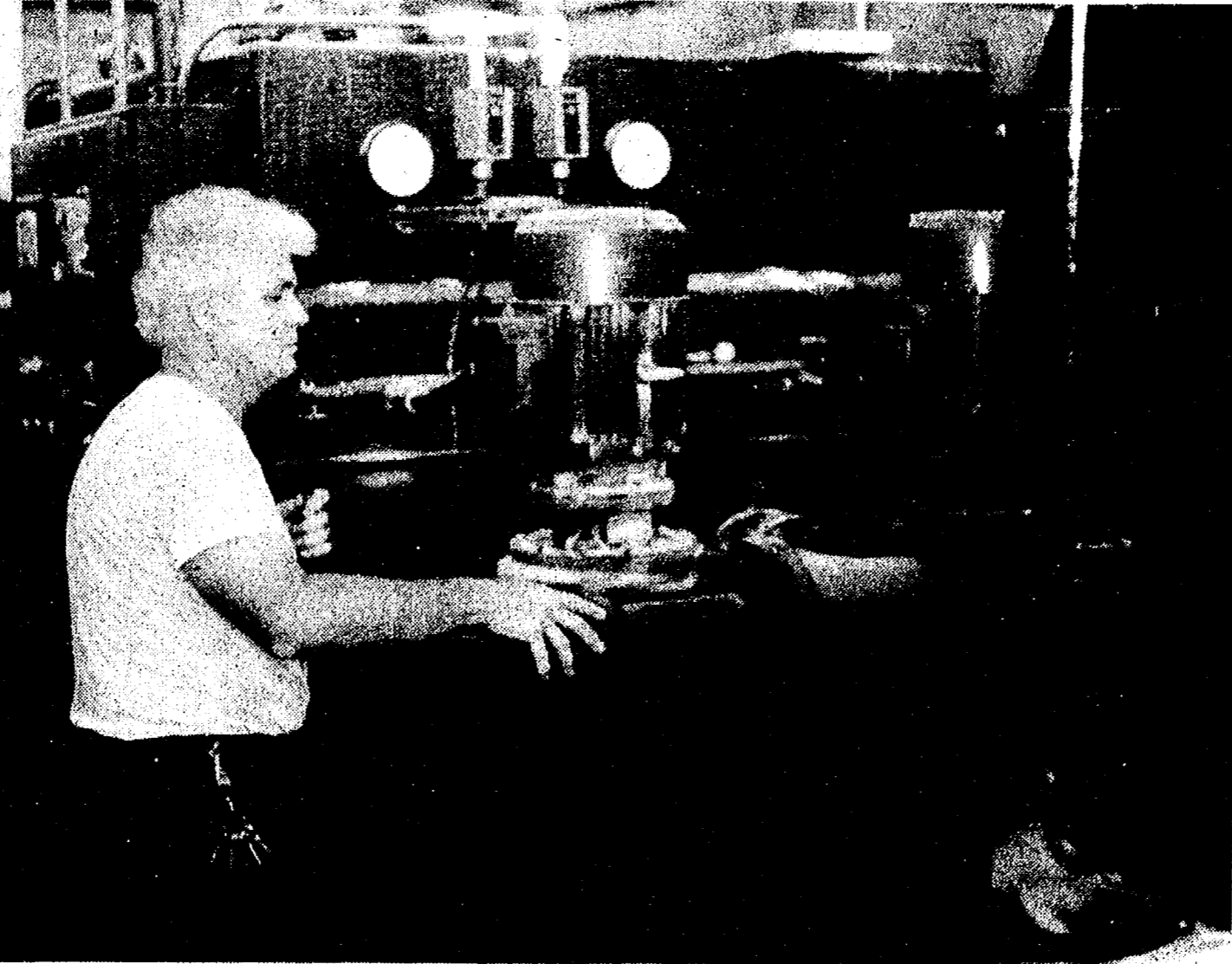
TOM McNAMARA , maintenance supervisor of the Charles S. Cameron swimming pool at Chelsea's Beach Middle School, inspects the twin motored filter which processes and recirculates 500 gallons of water per minute. Water in the pool
