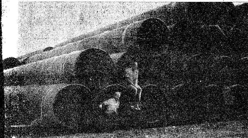
FOR THE PIPE LINE: These four-foot pipes, 10 feet long and 1/2 inch thick were made in one of Japan's large steel mills and shipped over to Valdez. Turner says that more than 400 miles of pipe are
